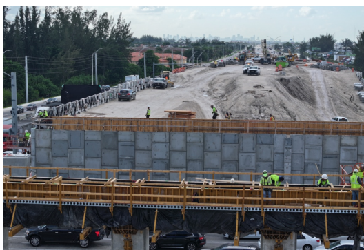
SR 25/US 27/Okeechobee Road at the NW 116 Way Intersection
